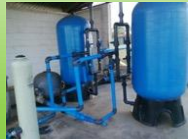
Rehabilitation of the Swaziland Railways water Treatment plant
