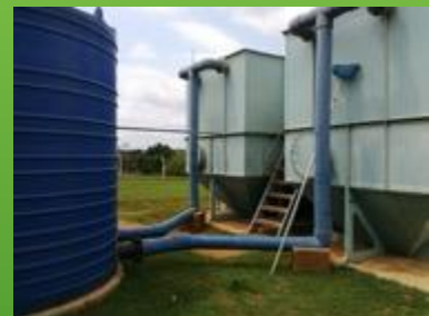
Rehabilitation of the 1.8 mega litre Potable water treatment plant for SWSC at Siphofaneni
